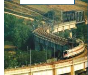
Alstom France Train Control Systems
