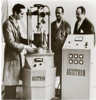
1954 One of the first EDM die sinking machines
